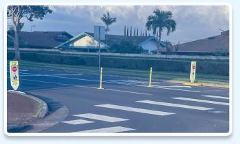
In January this year, a new gateway was installed by the City along Lanikuhana Avenue and Makaimoimo St. behind Walmart to help slow down drivers and protect pedestrians in this uncontrolled crosswalk. The poles are made of plastic, with retractable springs that are made to be hit and pop back up. Please watch out for pedestrians and drive safely!
